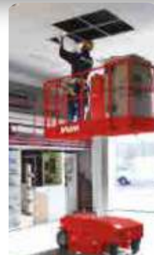
Installation and finishing work
